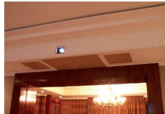
Porthole in bulkhead with projector behind
