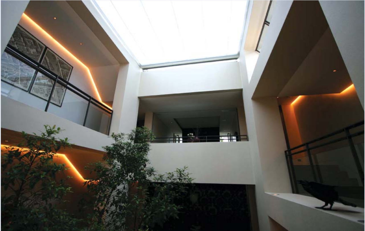
The motorised glass roof that helps control the temperature within the house.
